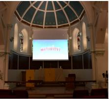
Motorised long drop screen allows the screen to be dropped to two operating heights – for main Chapel services and for the popular cinema club. The system also shows Freeview TV channels and has flexible inputs for instruments, laptop and microphones. A truly discreet and flexible AV system.
